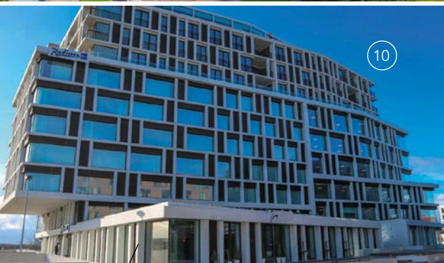
8. AL RAYYAN COMPLEX -TERTIARY AND RESIDENTIAL UNITED ARAB EMIRATES (OPRO+ WATER HEATER) ATLANTIC
